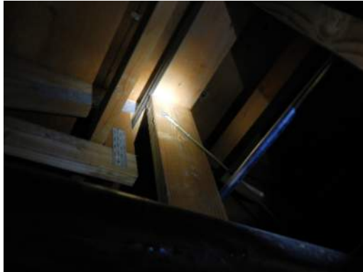
DISCONTINUOUS BOTTOM CHORD OF TRUSS
