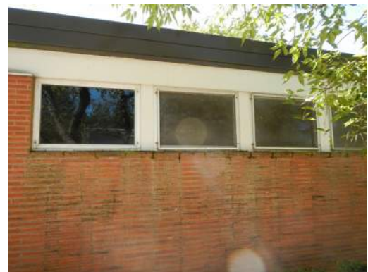
WATER DAMAGE IN BRICK VENEER
