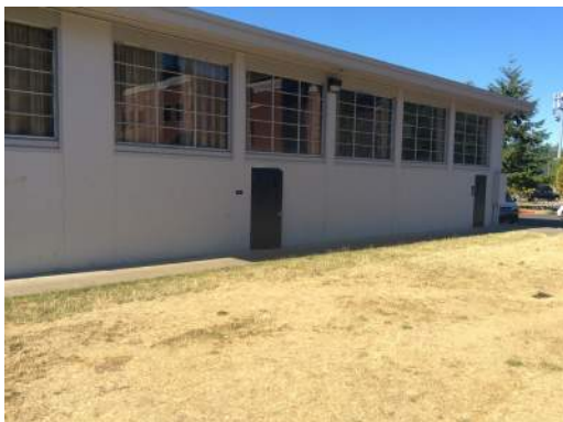
LACK OF LATERAL SUPPORT AT BUILDING END
