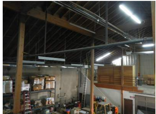
UNBRACED PIPING
