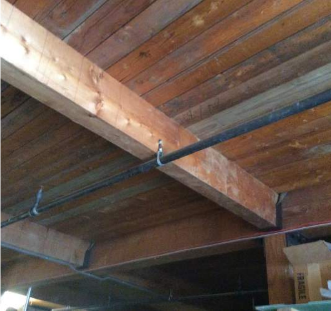
REMOVE STRAIGHT SHEATHING
