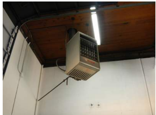
UNBRACED EQUIPMENT
