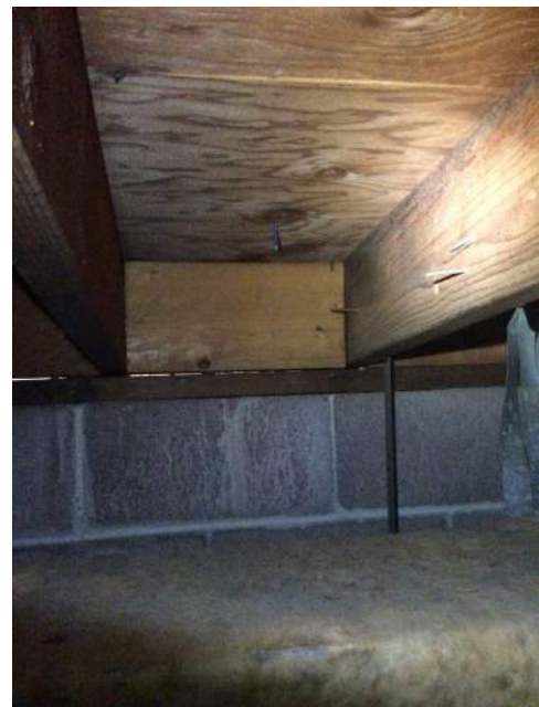
INADEQUATE JOIST CONNECTION
