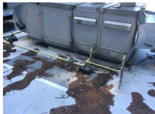
HARD CONNECTED GAS LINE
