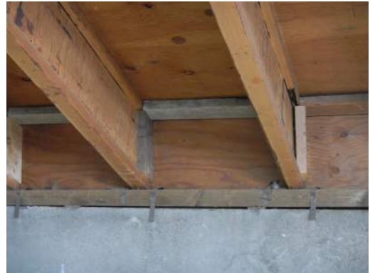
INADEQUATE DIAPHRAGM CONNECTION
