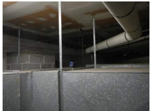
UNBRACED PIPING
