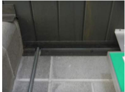
MISSING DIAPHRAGM CONNECTION TO LEDGER
