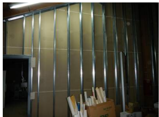
WALL NEEDS BLOCKING AND STRAPPING
