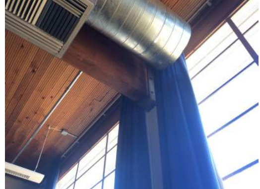
LACK OF SEISMIC CONNECTION AND BEAM SUPPORT
