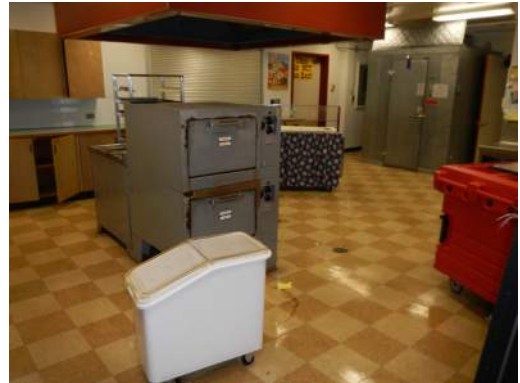
UNANCHORED EQUIPMENT IN KITCHEN
