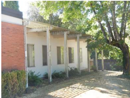
DETERIORATED TRELLIS
