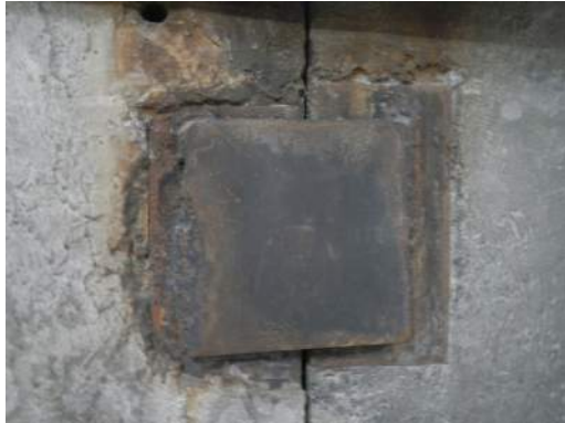
CORROSION IN PANEL CONNECTIONS
