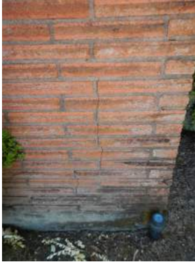
CRACKING IN BRICK VENEER
