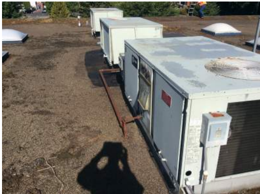
HARD CONNECTED GAS LINES
