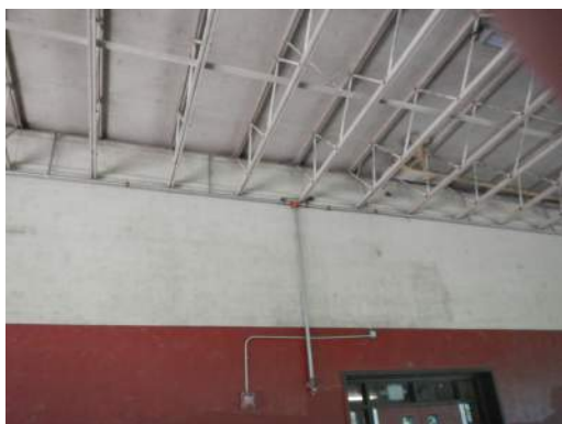
INADEQUATE DIAPHRAGM CONNECTION
