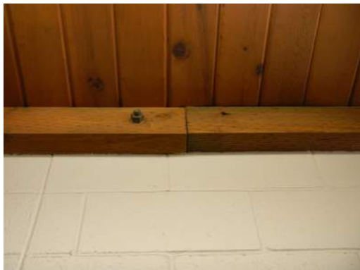
MISSING BOLT IN LEDGER
