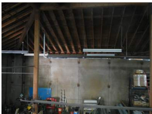
PENDULUM LIGHTING
