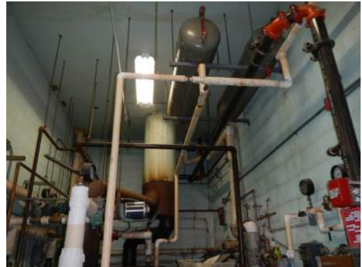
UNBRACED PIPING
