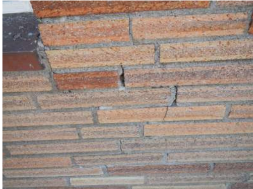
CRACKING IN BRICK VENEER
