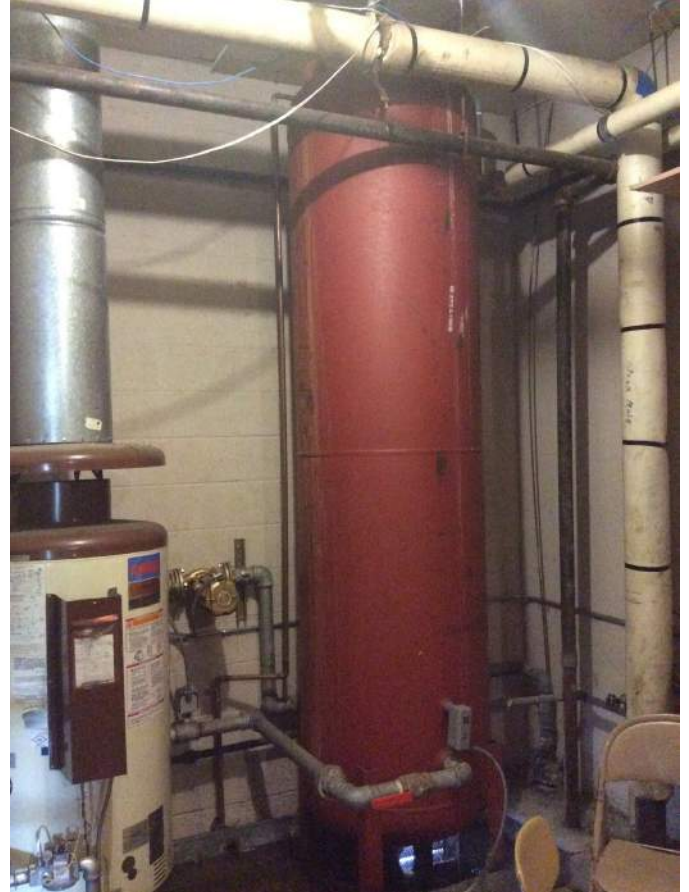
TANK TO BE BRACED FROM WALL
