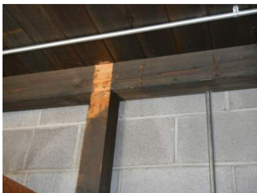
MISSING CONNECTION HARDWARE
