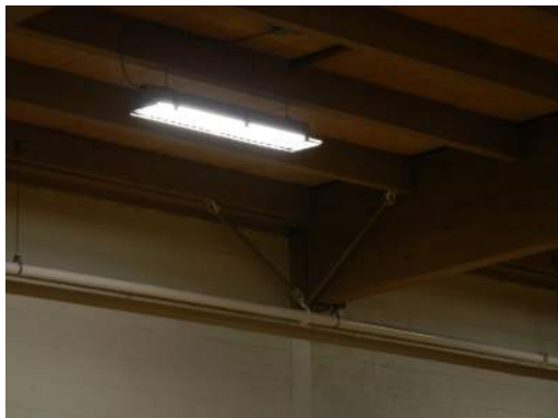
CROSS-GRAIN BENDING INDUCED IN JOIST
