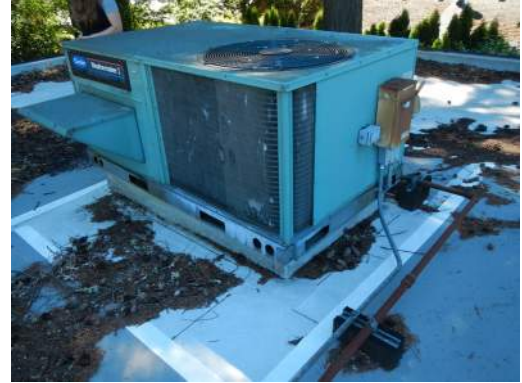
INFLEXIBLE MEP CONNECTIONS
