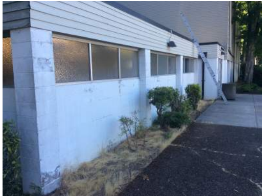
LACK OF LATERAL SUPPORT AT BUILDING SITE
